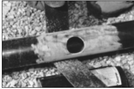
Fig. 4. Abrade all bonding surfaces on the pipe with emery cloth or a flapper sander.
